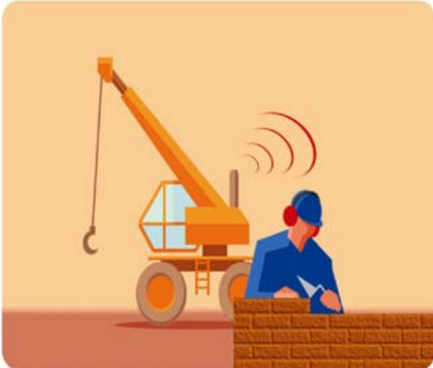
Figure 5.13 A worker uses ear-muffs attached to his helmet at a workstation where head protection is required
